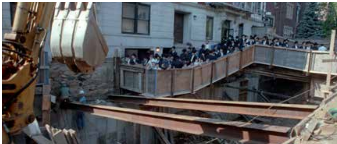
Chassidim wait on line to pass by the Rebbe while construction takes place, Elul, 5751.
